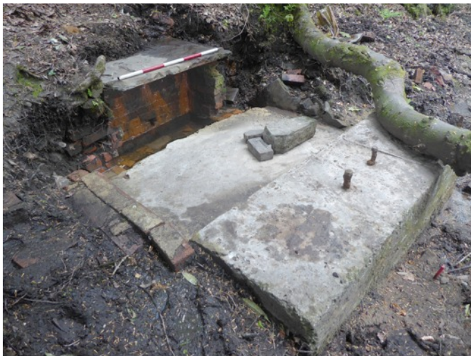
The bridge support with two large iron bolts which would have secured the walkway.
