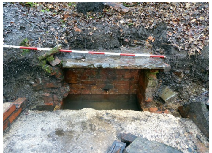
The spring area is housed within the brick structure with a flagstone cap. Water enters through the back wall just above the water line and collects in a concrete tank.
