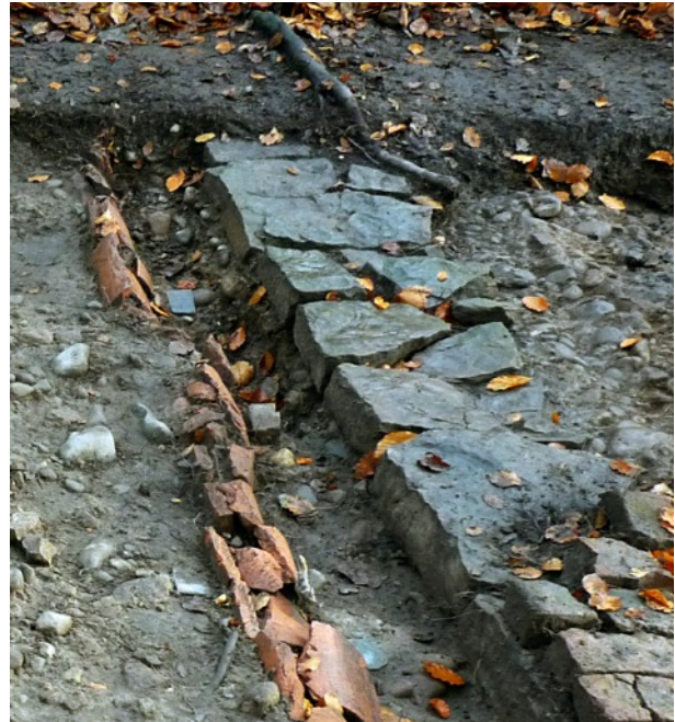
Western foundation of north wall. 40 cm wide using irregular flagstones.
