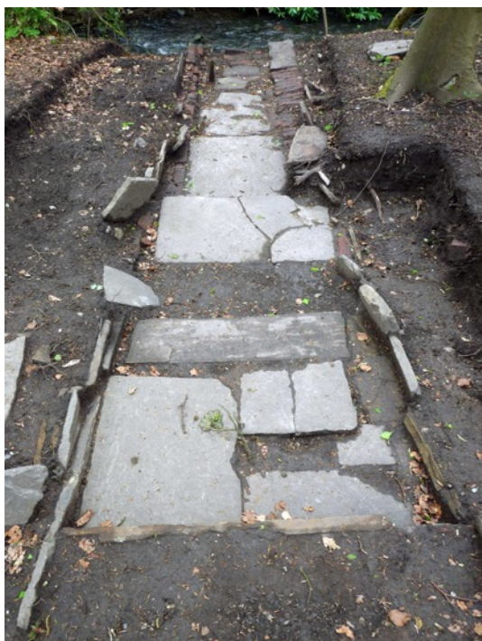
Looking north towards the Trub Brook. The footbridge path is constructed from reused paving stones edged with brick at the northern end. Vertical flagstones prevent garden soil spilling onto path.
