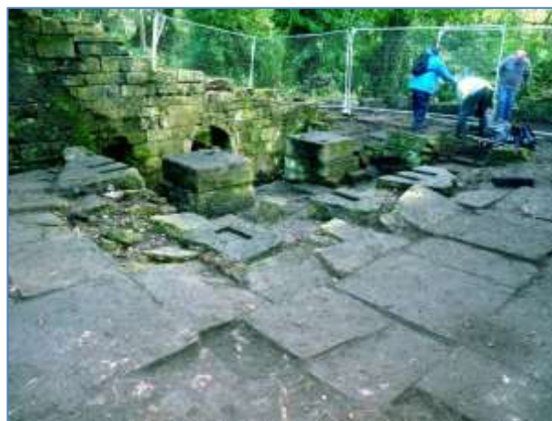
Figure 3 Western face of wheelpit wall and supports for branch tree
