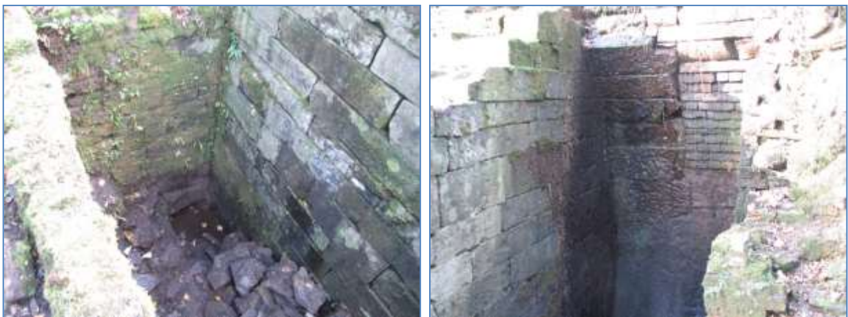
Figure 5 wheelpit south showing tailrace, wheelpit north showing expansion work
